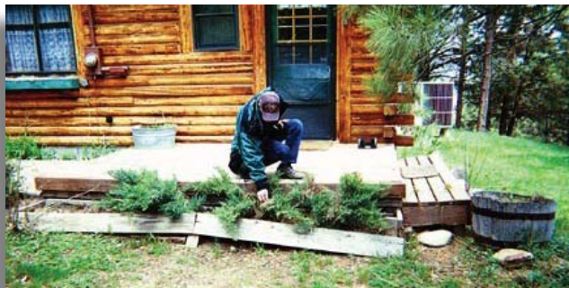
Flammable vegetation in direct contact with house
